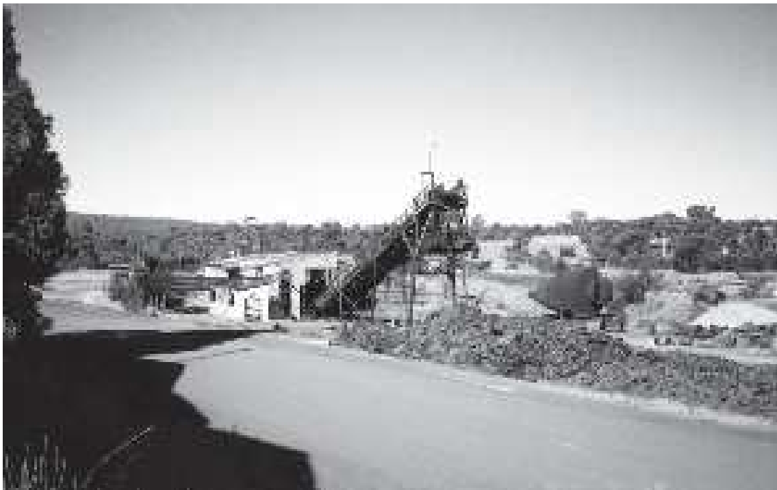
Wundowie Timber Mill in 1991 – 12 years after its closure – showing the waste timber that was used as fuel in the retort to make high quality iron.
